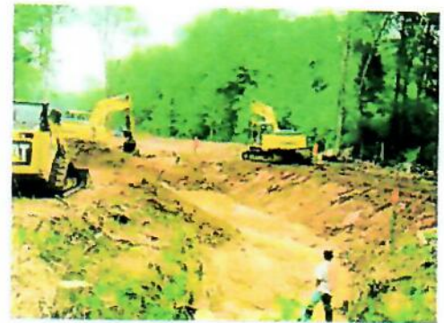
A creek during restoration.
